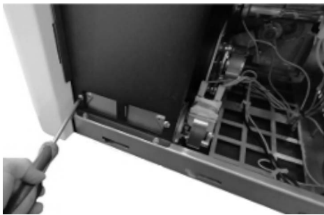
Fig. 78 - Reinigung Raumventilator (Atena 3 Plus 12/14 - Duke 12/14 At - Saba 12/14)
